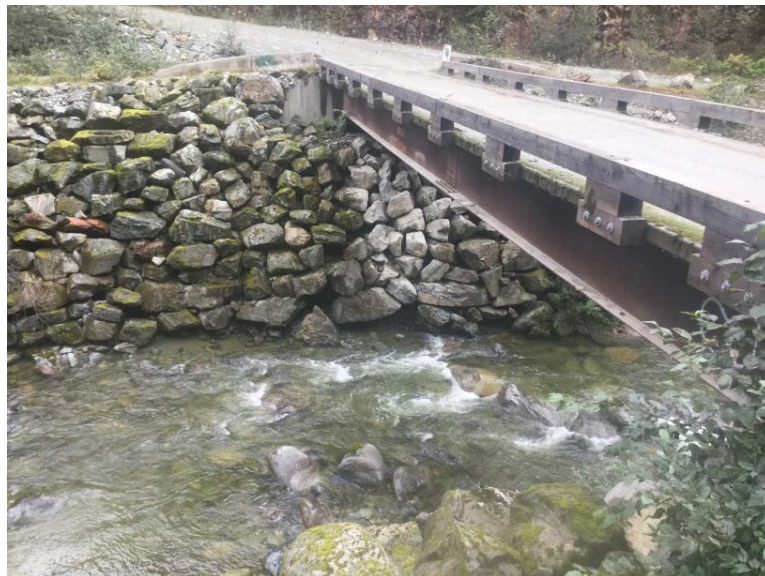
Right Bank Abutment when facing downstream
