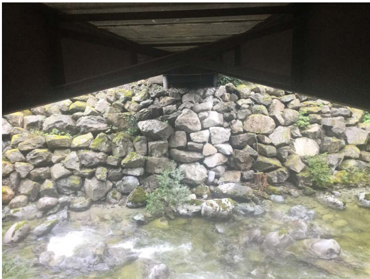
Left Bank Abutment when facing downstream
