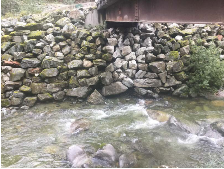
Right Bank Abutment when facing downstream
